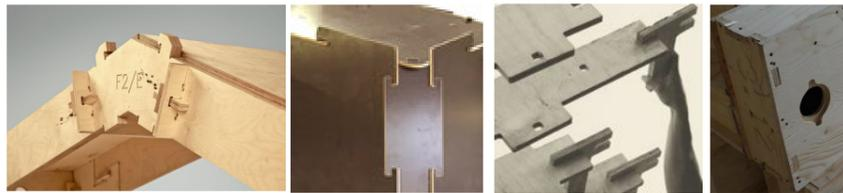
*Figure 1: Diverse project details using friction-fit plywood*
