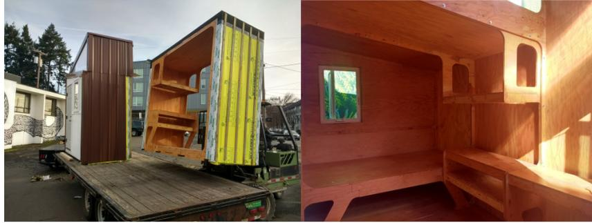
*Figure 8: Programmatic units of the PlyPAD, in transport and assembled*
